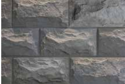
Step 3: Use the same color grout for the grouting, and to cover the nail edges.
