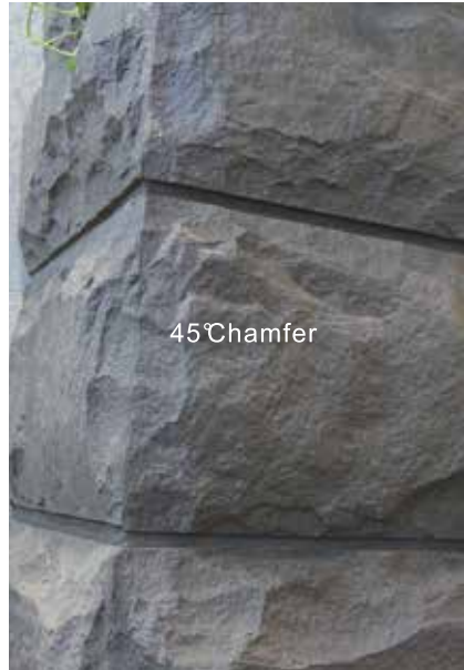
External Corner: Installing with the whole piece, 45° Chamfer, using the same color for grouting.
