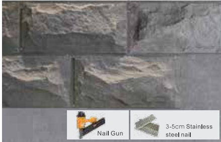
Step 2: Put stainless steel cement nails at the four corners and middle edges of the product.
